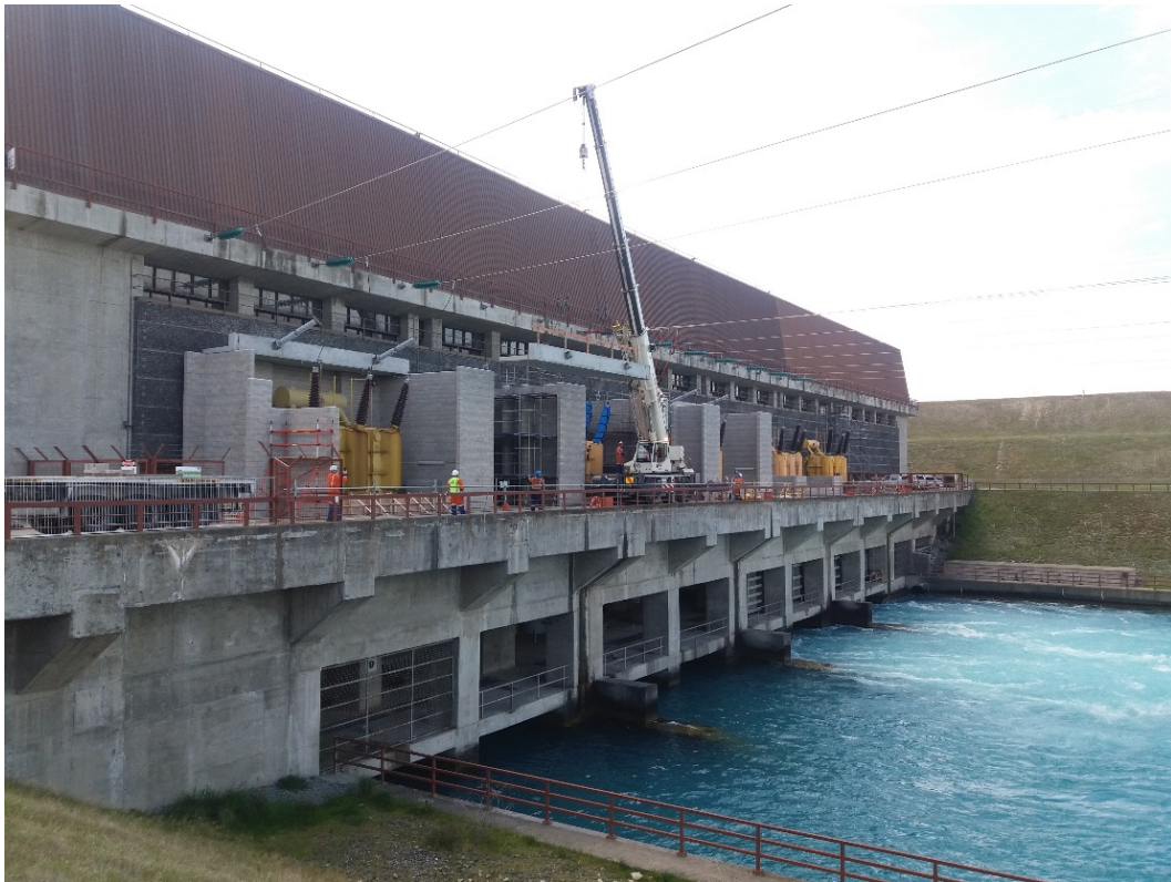
Figure 11: Pre-cast canopy installation
