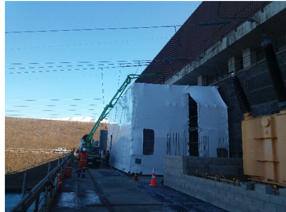
Figure 8: Wrapped scaffolding
