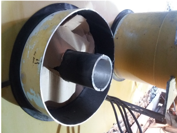
Figure 14: Cut IPB enclosure and busbar
