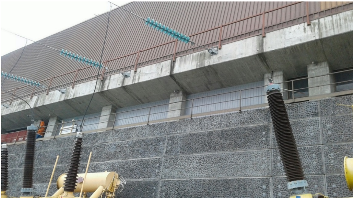
Figure 16: Completed Speedwall® window protection showing transport trolley on left
