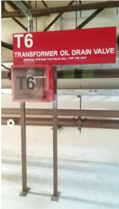
Figure 12: Emergency oil drain valve
