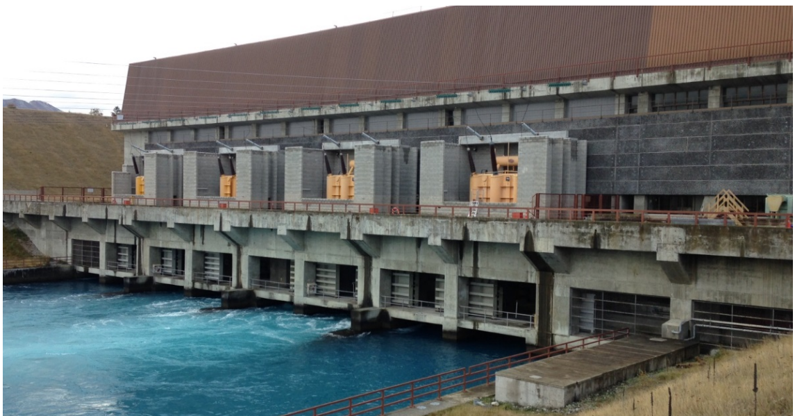
Figure 2: Ohau A transformer platform after project
