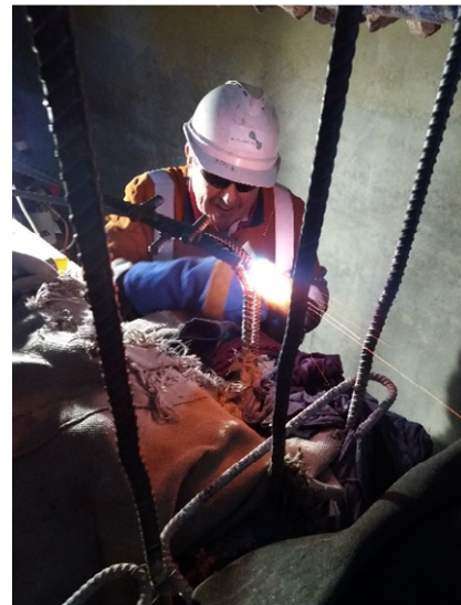
Figure 10: Re-bending with heat
