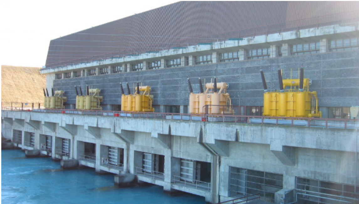
Figure 1: Ohau A transformer platform before project
