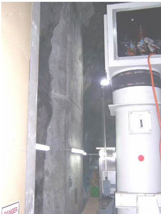
Vault Before – cable riser shaft behind concrete wall on left
