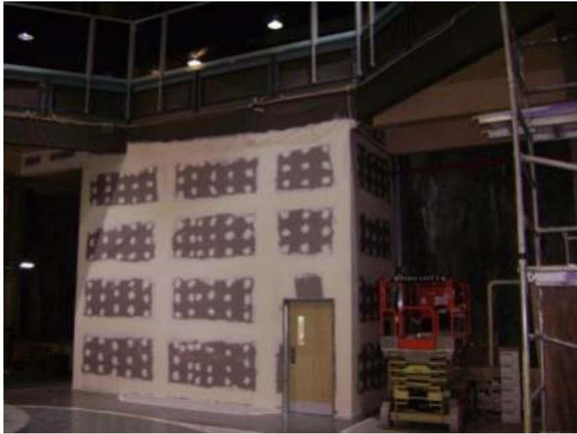
Figure 7 Manapouri Power New Stair Enclosure Machine Hall level – before completion
