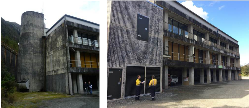
Figure 4 Manapouri Power New Ventilation Building Before and After Construction
