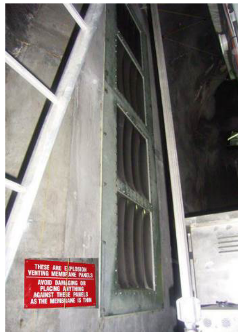
Vault Vents installed
