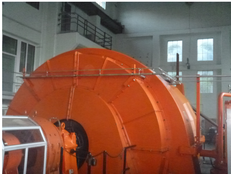
Figure 4: Nitrogen and mist discharge piping and entry.
